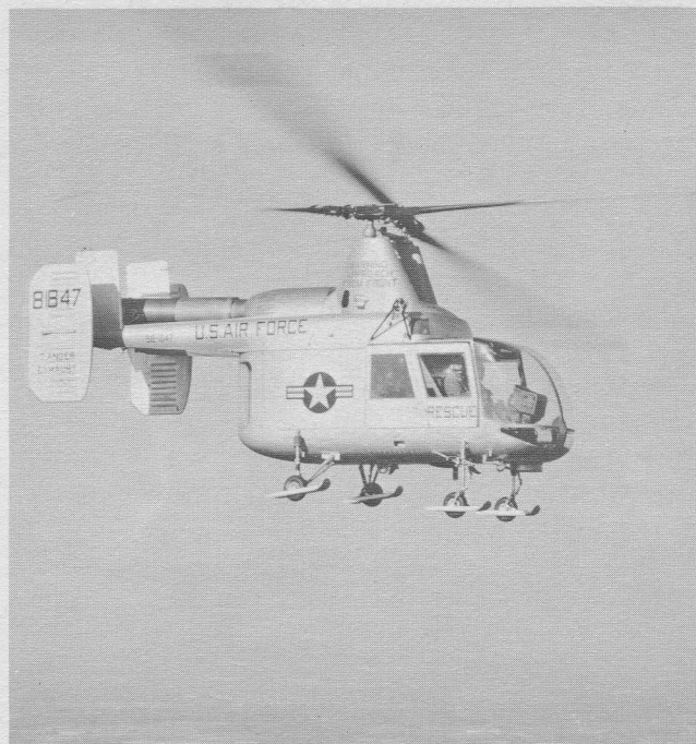
H-43B — Designated the HUSKIE, turbine powered aircraft of this type are now being delivered to the Air Force.
