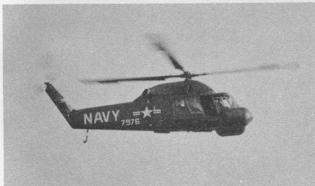
SEASPRITE MAKES FINAL APPROACH for water landing with emergency flotation bags inflated.
