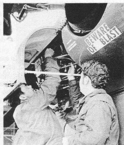
In photo, left, AMS3 Miller, assisted by AW1 Holder, removes a main rotor blade and retention assembly as LCdr Hilgeman and AA Murphey observe. In second photo, right, ADJ2 Auguston instructs ADJ3 McKenna on troubleshooting the fuel control actuator. (USN Photos)
