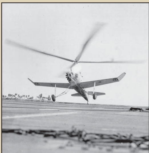
Taking a trap? Heck, no! The Pitcairn XOP-1 lands aboard USS LANGLEY (CV-1) during evaluation. Unable to hover its usefulness was limited for fleet operations. (NMNA)
