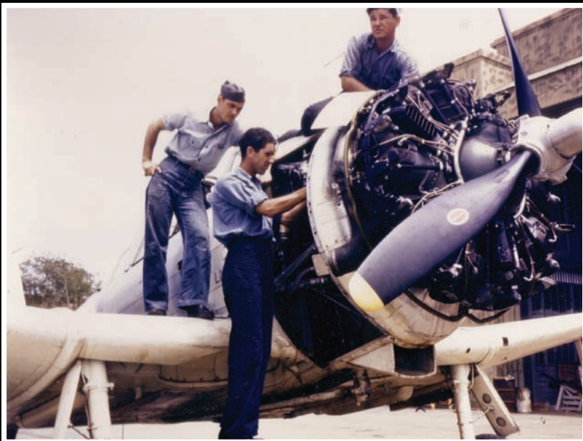
Sailors tend to the engine and accessory section of this Douglas SBD-5 Dauntless at a Caribbean air base after an ASW patrol in 1944. The Chief Machinist Mate is supervising the work. Engine is a Wright R-1820 "Cyclone". (NHHC)
