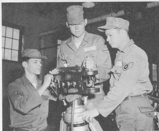
A2/c James Wells and A2/c Scott Vandenburg listen attentively as S/Sgt. Andrew Cota gives them instruction on the proper way to perform an azimuth bar runout check.
