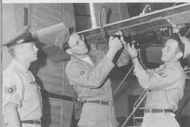
ELEVATOR RIGGING —SSgt. Wilder, Instructor; A2C Morphis, Grand Forks AFB, N.D.; A1C Alexander, Charleston AFB, S.C. (USAF photo)
