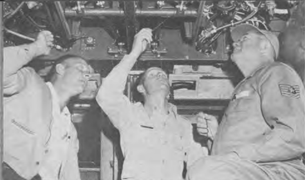
COLLECTIVE THRUST BEARING HEIGHT SETTING —Mr. Kenyon, Instructor; Mr. Hawkins, Kirtland AFB, N.M.; TSgt. Perkins, Spokane Intl. Aprt., Wash. (USAF photo)
