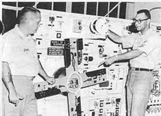
THE ROTOR DE-ICING system of the HU2K is discussed by Chief MacCracken and Glaeseman.
