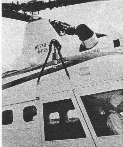
The rescue hoist is located on the right side, immediately behind the pilot. The winch can be operated by pilot or crewman.
