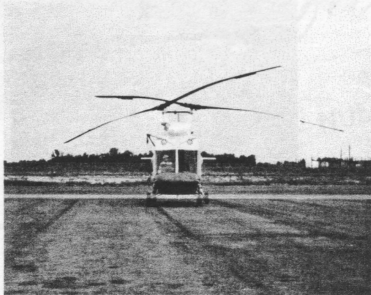
The front view clearly shows the forward engine installation, electronics chin pod and rescue hoist.
