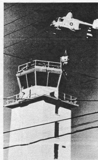
HERE TO THERE —Civil Engineering, Maintenance and Supply Groups teamed up with an HH-43B crew at Stead AFB, Nev.; in placing this 700-pound beacon atop the new control tower so the light would be back in operation by nightfall. Aboard the HUSKIE were Maj Harold Wheeler, pilot; Capt William L. Henderson, copilot; and SSgt Roger Winkle, crewman. (USAF photos)
