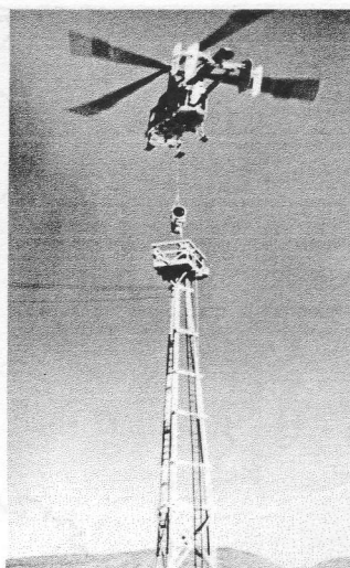
HERE TO THERE —Civil Engineering, Maintenance and Supply Groups teamed up with an HH-43B crew at Stead AFB, Nev.; in placing this 700-pound beacon atop the new control tower so the light would be back in operation by nightfall. Aboard the HUSKIE were Maj Harold Wheeler, pilot; Capt William L. Henderson, copilot; and SSgt Roger Winkle, crewman. (USAF photos)
