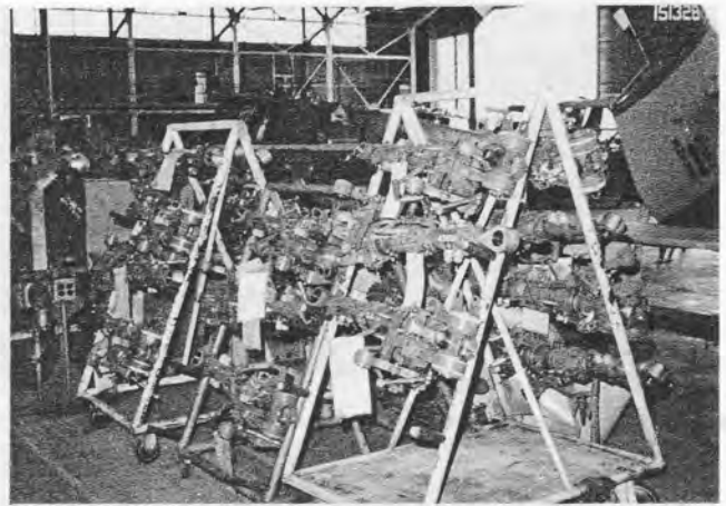
RETENTION OVERHAUL —Retentions awaiting processing to determine scope of work, PAR repair or overhaul.
