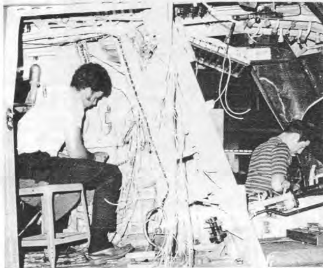
WIRING —Shown is a small portion of the three miles of wiring and harness assemblies being installed in the helicopter. The wiring from the roof line up is mostly independent of the fuselage wiring and is terminated by connectors which allow free access for completion of wiring transmission and engine areas.
