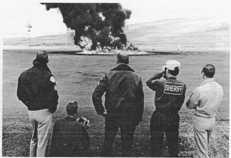
Southern California officials watch as Air Force HH-43, upper left, flies to burning wreckage with 1000-pound Fire Suppression Kit. The unit is being flown to ground-based firemen who will use the light water foam in the FSK to clear a path through the flames. The helicopter's rotor downwash is also used in suppressing the fire. The billowing black smoke in this picture will soon be eliminated as the Air Force changes to smokeless fire, using water sprays for fire-suppression training. Left to right are, Sgt David McGill, Los Angeles Police Department; Deputy Joseph Bator, Sgt Roger Griessel, Lt Robert A. Morse, San Diego Sheriff's Department; Sgt Cliff Owens, Los Angeles Police Department.
